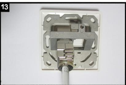
Assemble the first Keystone Jack with snap in operation in the metal frame.
